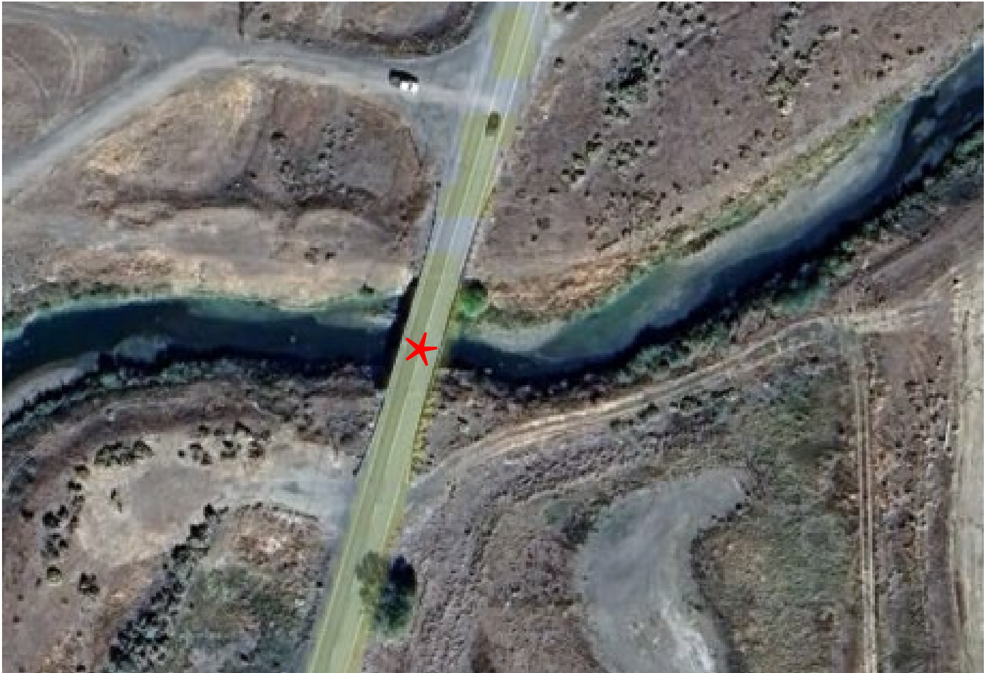
COUNTY ROAD 54 BRIDGE - NORTH FORK PIT RIVER
